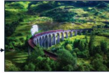
Glenfinnan Viaduct, Inverness-shire, Scotland
